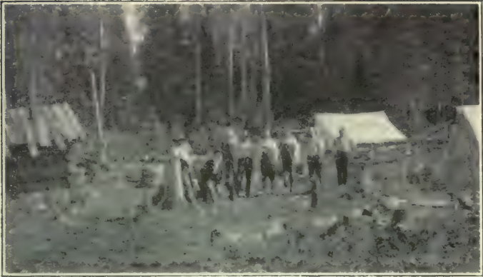
A Road-gang in the Clay Belt—Good bush roads are a prime necessity in early settlement.
